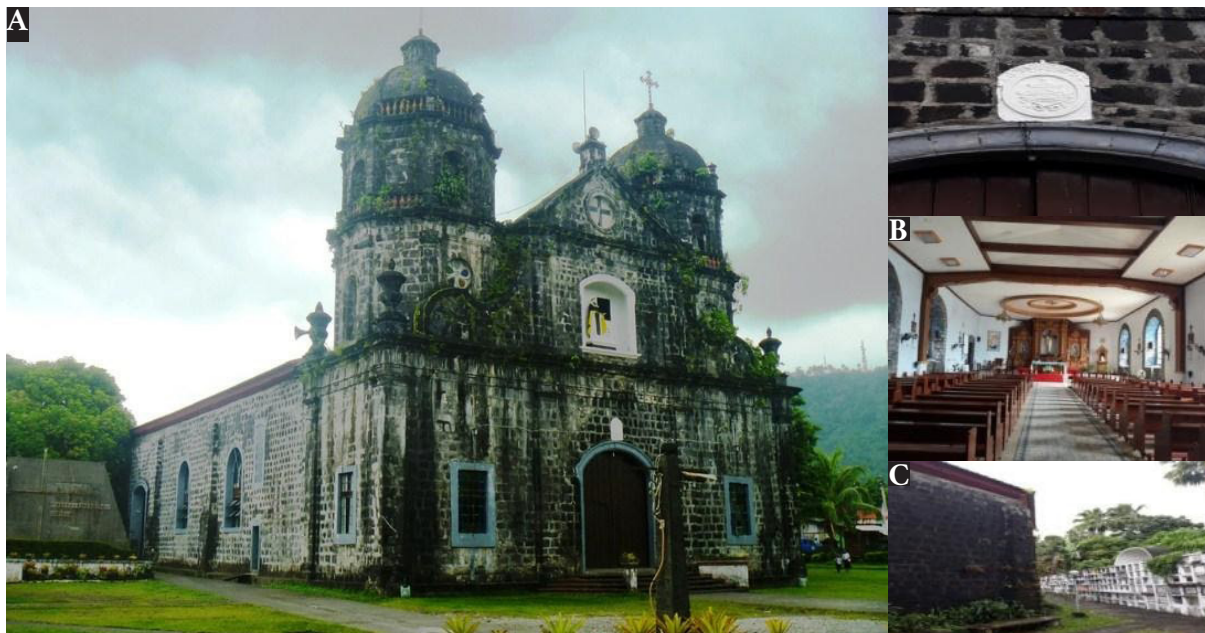
Figure 2. St. Dominic de Guzman Church and its stone walls (A), interior (B) and cemetery (C).
